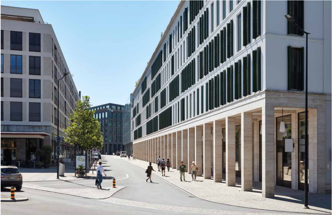
↑ Figure 3. Arcade street, view from the station. Ricti Quartier, Wallisellen (Photo: Maximilian Meisse).
