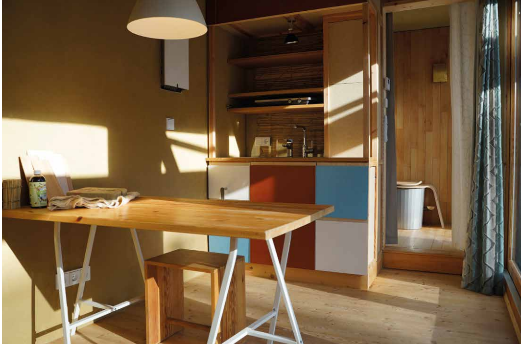
↑ Figure 2. The interior of Zero Waste Space is designed as a fully equipped, autonomous working and living unit. In the kitchen area, a degradable kitchen system consisting of a wooden construction with straw hemp panels was tested (Photo: Tanja Lücker).
