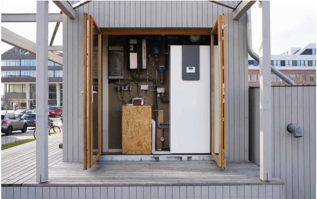
↑ Figure 5. The heart of the facility is its own technical unit, which controls the water, electricity and heat supply (Photo: Tanja Lückert).
