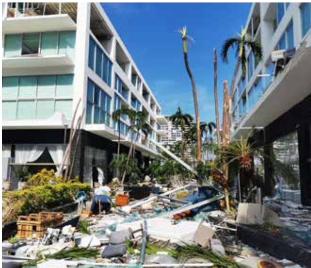
The damage caused by Hurricane Otis in Acapulco, Mexico. © Jessica Rodriguez Leon/ Shutterstock
