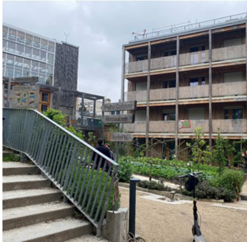
Figure 13. To the left, the greenhouse building with workshops. The building to the right contains 15 flats for homeless and 5 for students. Photo C. Gullström.
